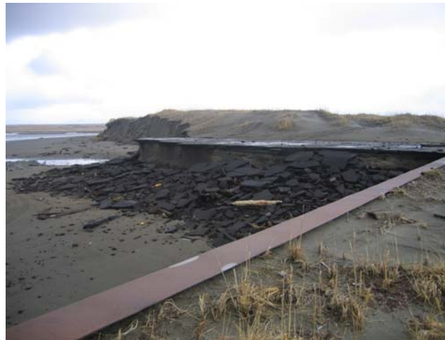
Photo 4: Sheet Pile Erosion Protection, following October 2004 Storm.
