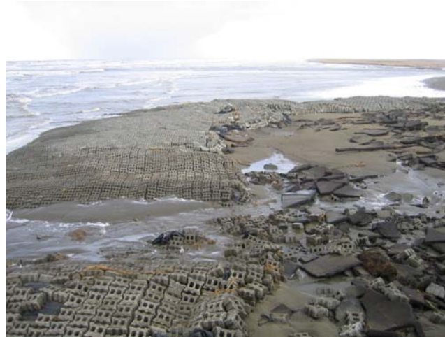
Photo 2: Failed Interlocking Concrete Block Erosion Protection, following October 2004 Storm.
