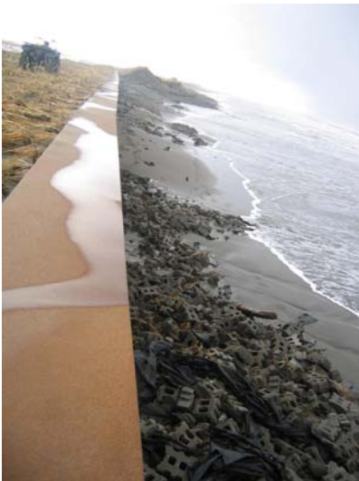
Photo 3: Sheet Pile Erosion Protection, following October 2004 Storm.
